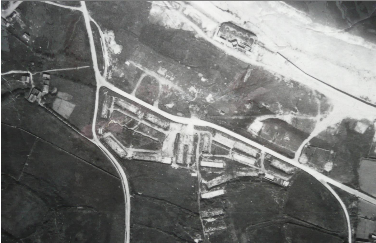
Helgoland Camp from the air showing hut bases and internal roads, after it had been dismantled. The beach depot can be seen to the north. (1949)
