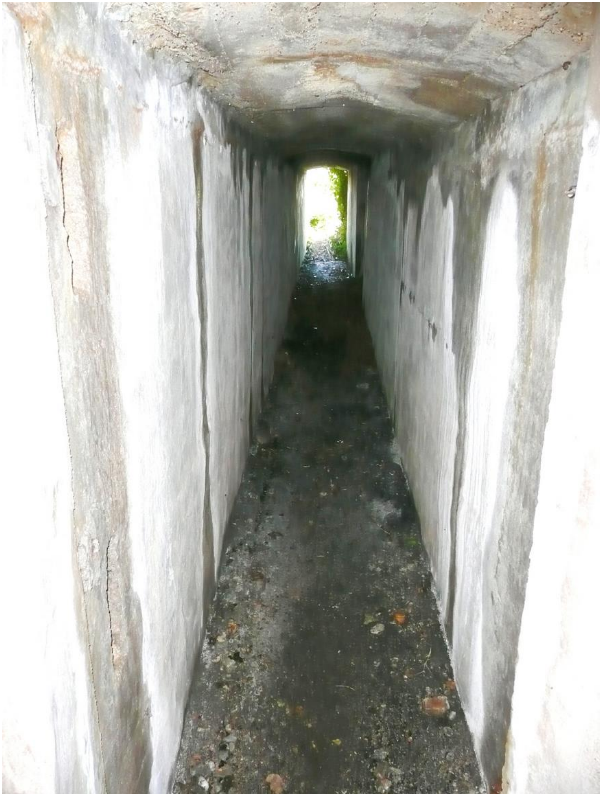
The Sylt tunnel looking back towards its exit to List's Chalet.
